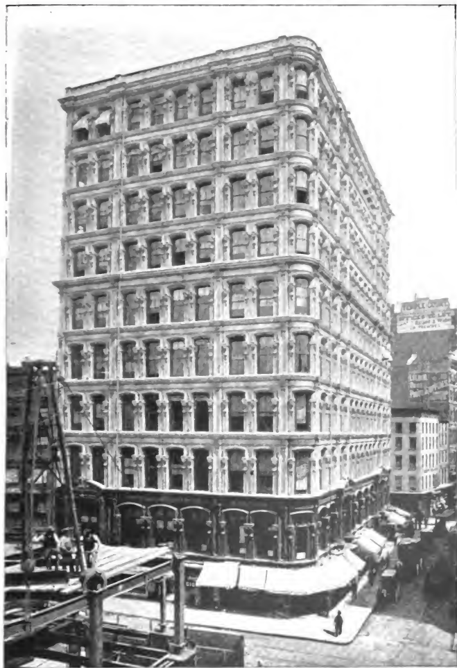
BENNETT BUILDING. NASSAU, FULTON AND ANN STREETS.
